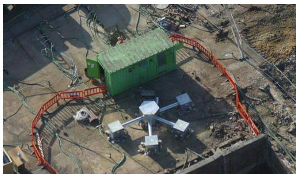
**Figure 1.** Arrangement for RF heating and thermal enhancement of soil vapor extraction at an industrial site in London (photo: Ecologia Environmental Solutions Ltd., Kent, UK).
