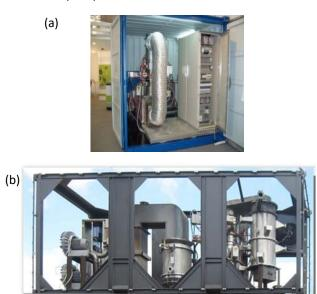
**Figure 5.** MOS reactors installed in 20-feet containers, with capacities of 600 m<sup>3</sup>/h (a) and 4500 m<sup>3</sup>/h (b).
